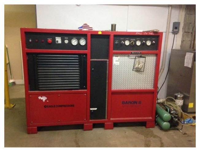
Breathing air compressor installed in lower level building 1 and AC electric connected
